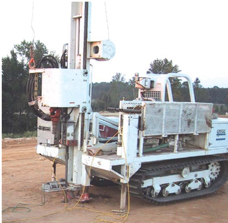
Figure 12 Small anchored drill-rig unit
